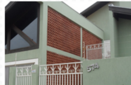
Walls and decoration
